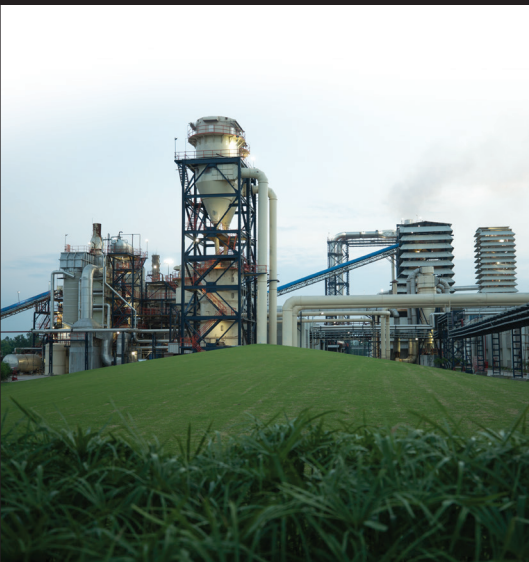
View of MDF Plant, Hoshiarpur, Punjab
